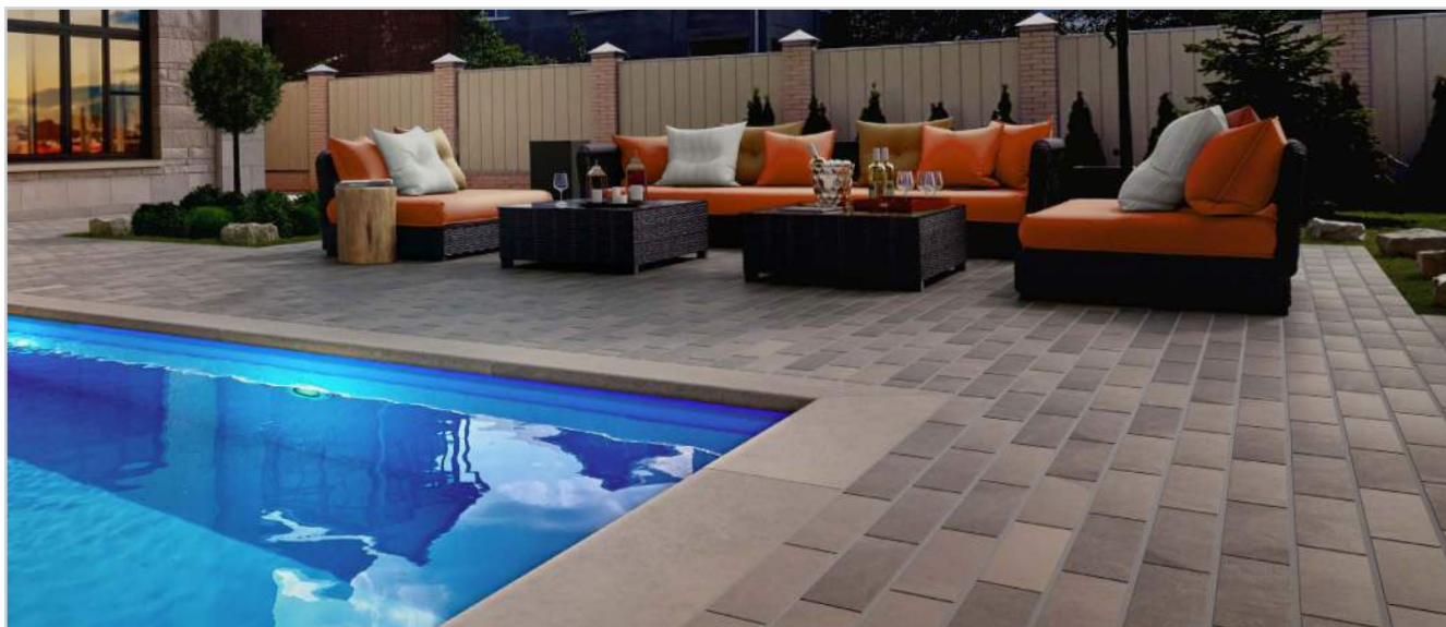
Plank pavers in running bond pattern with pool coping.
