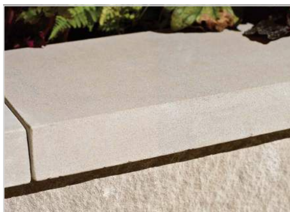
Sill used as a smooth edge wall cap.
