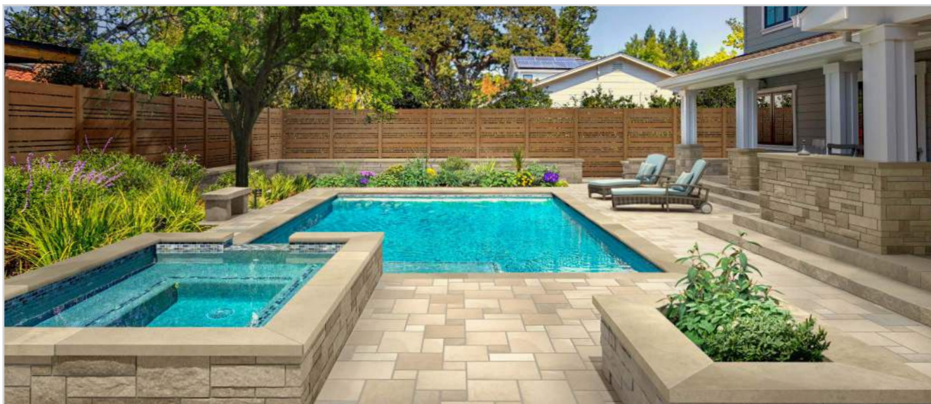
Small format pavers in the Lyon pattern (traditional French) with pool coping, smooth sills as wall caps, and 3" and 6" garden wall.
